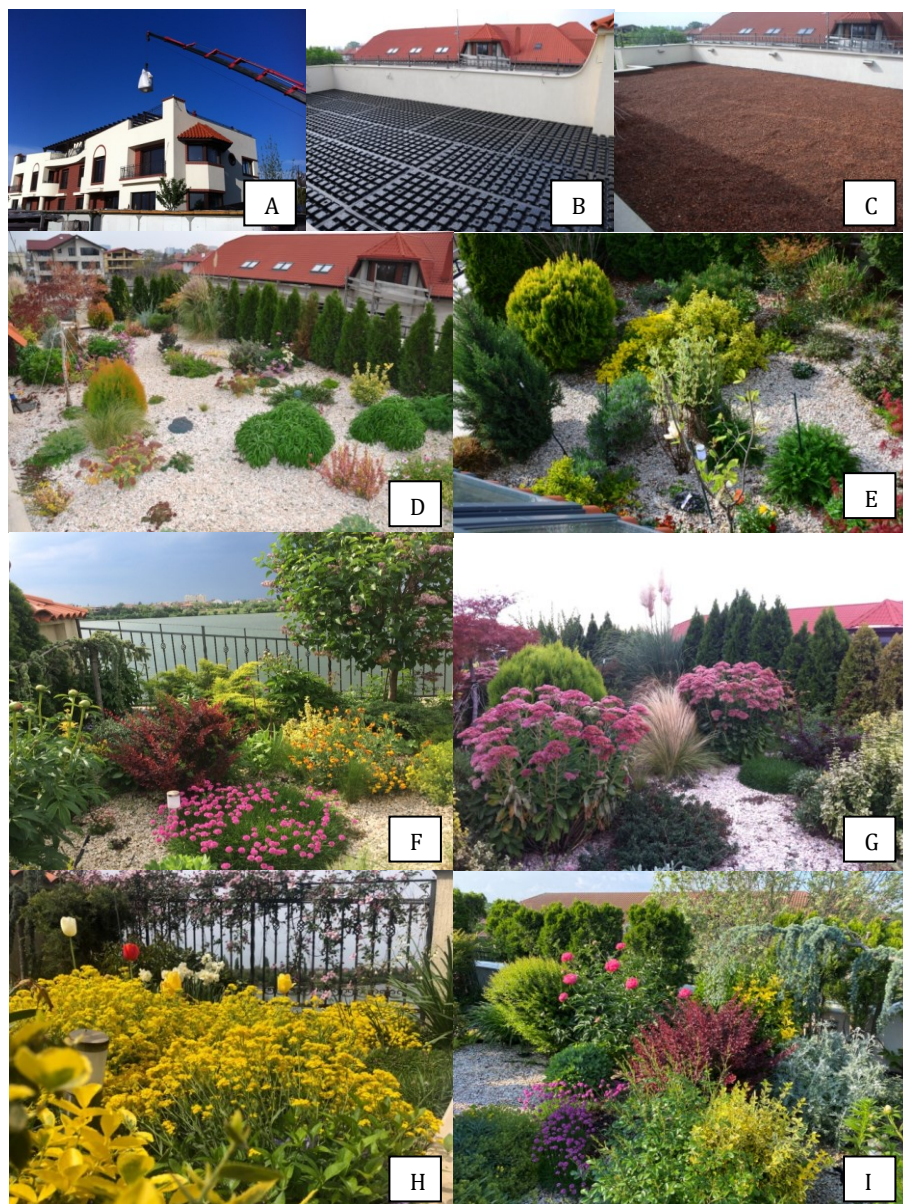
Fig. 1. Progressive development of the rooftop garden across years: A - location of the terrace, B - drainage layer of the terrace (2011), C - substrate layer of the terrace (2011), D - vegetation in 2013, E - vegetation in 2016, F - vegetation in 2019, G- vegetation 2021, H - vegetation in 2022, I - vegetation in 2023.
